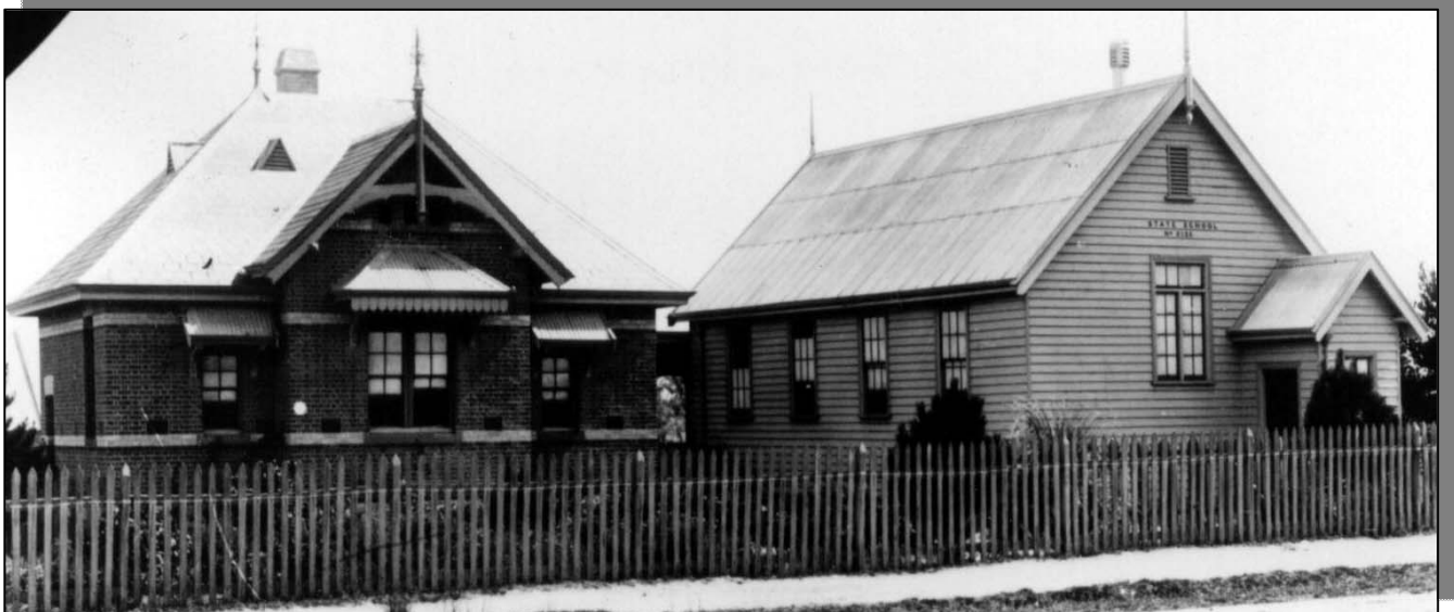
An early photograph of Morwell School (No.2136) with residence at left
