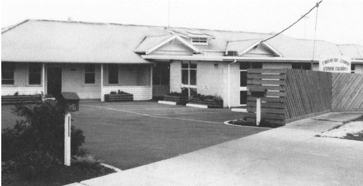
Morwell and District Community Hospital
