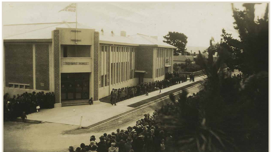
Opening of the new Town Hall on the corner of Commercial Road and Hazelwood Road - known as O'Rourke's Corner - on Tuesday 27 October 1936
