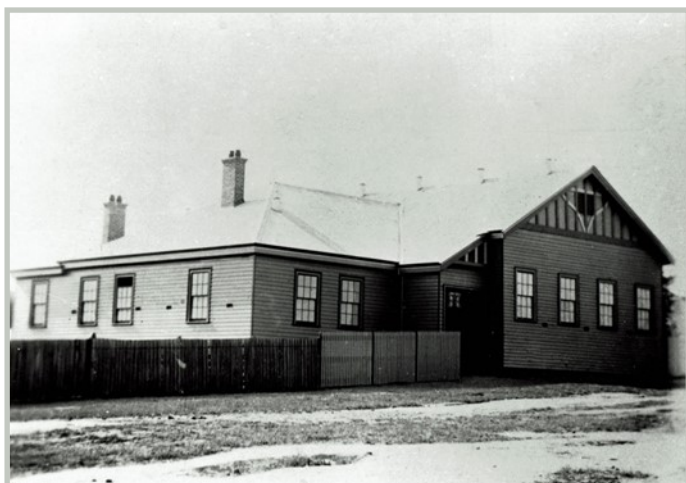
Mechanics' Institute facing Tarwin Street
