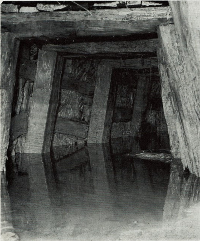
Entrance to the drive shaft that connects with main vertical shaft. The water was in process of being drained when this photograph was taken.
