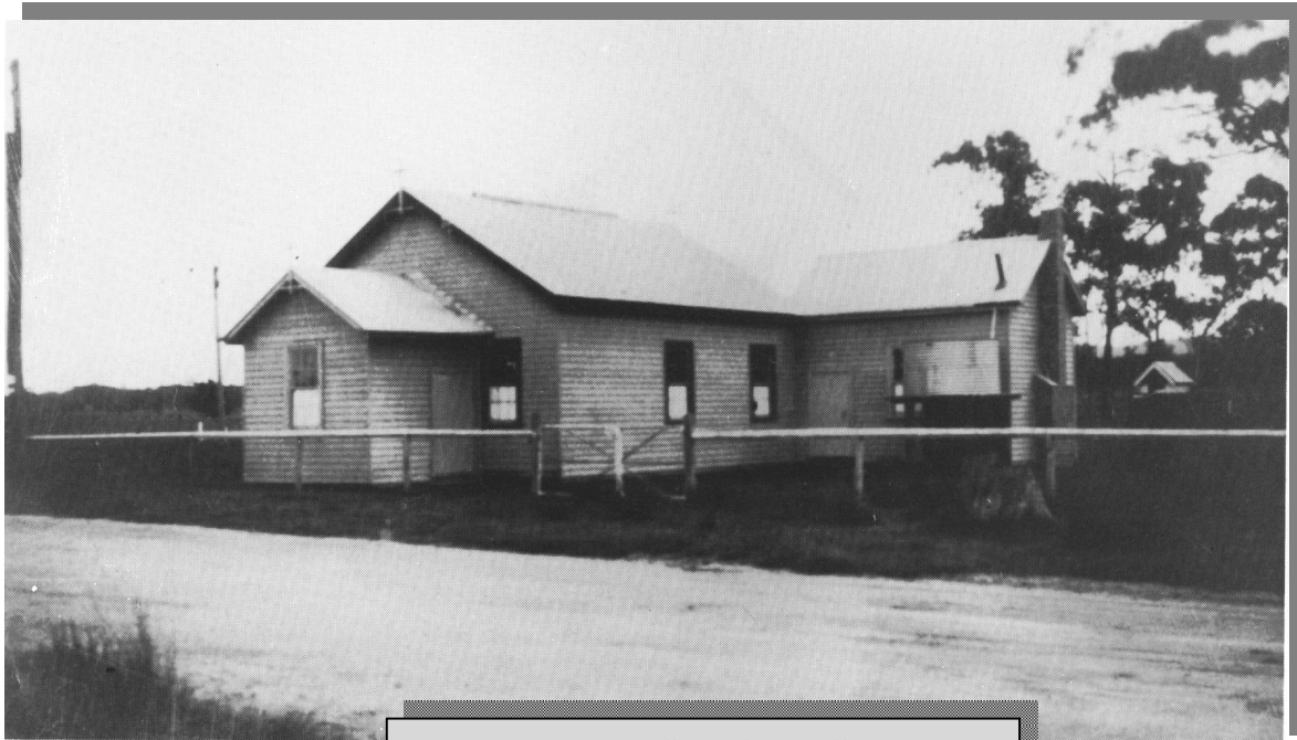
Morwell Bridge Hall
