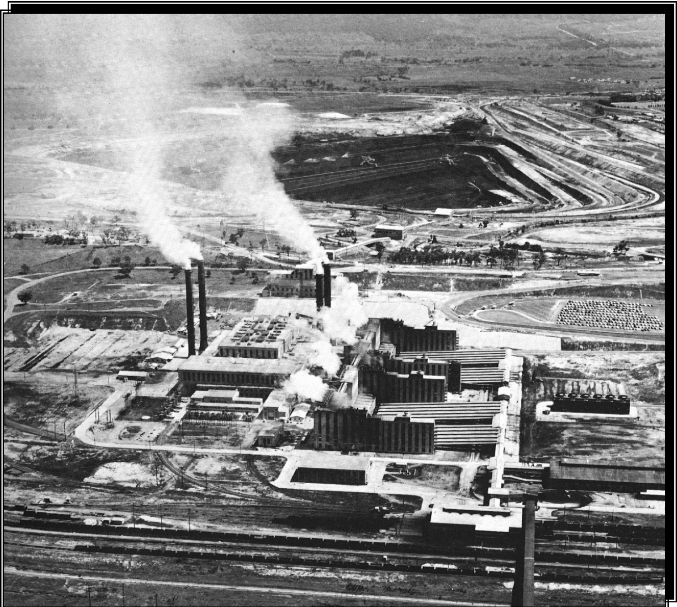
Morwell Briquette & Power Morwell Open-Cut in Background
