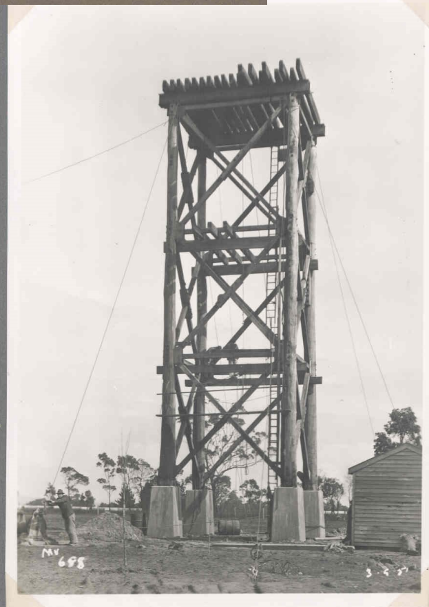
688 TRANSIT COTTAGES TOWER FOR WATER SUPPLY
